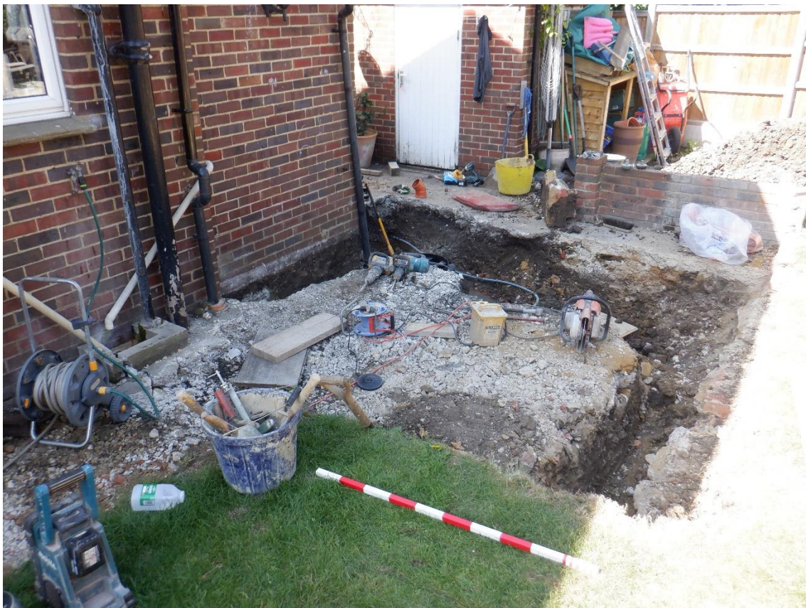
Plate 3. Ground reduction and trenching (looking SSW)
